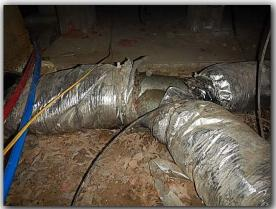
• AC vents should suspended from the floor joists and not be positioned on the ground. A substantial amount of cold air was entering the crawlspace. This is indicative of air duct leaks. Further evaluation and repair is I=Inspected NI=Not Inspected NP=Not Present D=Deficient
