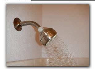
• The shower head in the down stairs bathroom has inadequate flow.
