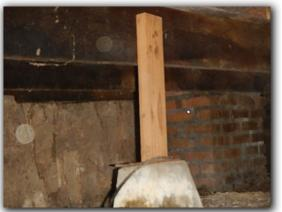
A 1X6 is being used as a pier support. Cement or 4x4 is recommended.
