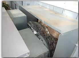
• The coil cover / louvers are missing and the supply and return ducts should be covered.
