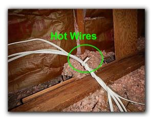
• Abandoned wiring should be replaced or appropriately terminated with wire nuts and protected in a junction box.
