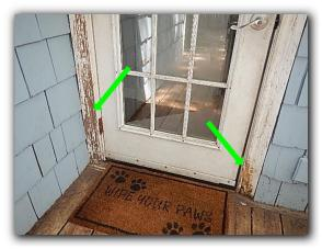
• Paint is needed to protect wood from water damage in the following location(s) rear door
