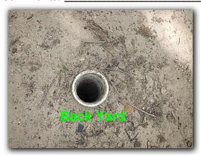
• Plumbing Clean-Out covers are damaged or missing. These should be replaced to prevent rodent, insect and reptile intrusion.
