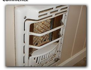
Gas Bathroom Wall Heaters are not vented to the exterior and should not be used. This is recognized as a safety hazard.
