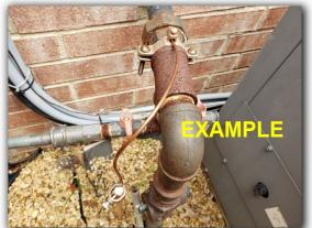
• The Gas meter or line should be grounded to the earth. (see EXAMPLE)
