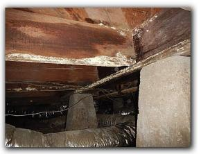
Moisture and damp soil was observed in the crawlspace. A white substance was observed on more than one floor joist. A substantial amount of air
