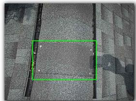
• Exposed nail heads were observed on the roof shingles. All exposed nail heads should be sealed with roofing caulk or sealant.
